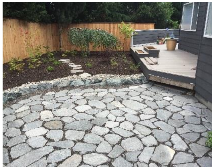
Above: HIP infiltration trench installed in 2016
