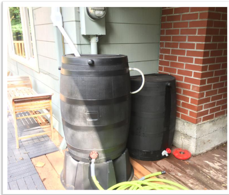
Rainwater harvesting system installed to water new native plants.
