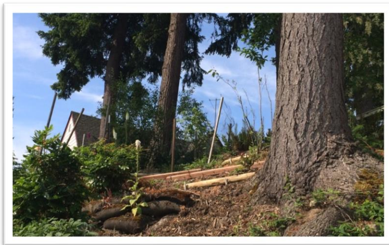
Half logs staked across a steep slope to hold new mulch in place.
